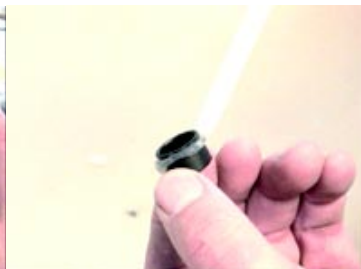
Run bead of quick adhesive around pin cap and place in hole.
